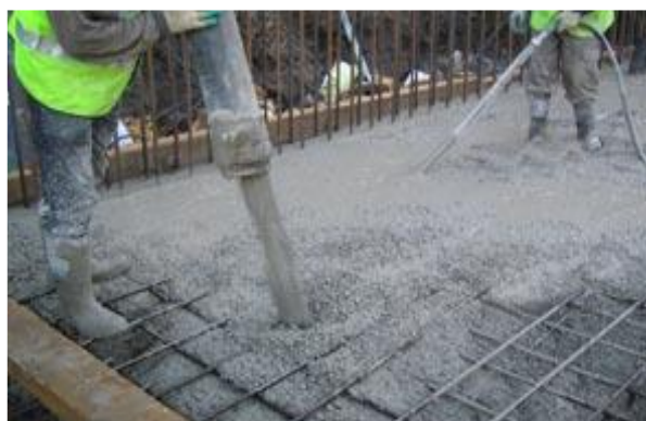
FIG NO 3: PLACING OF GGBS
