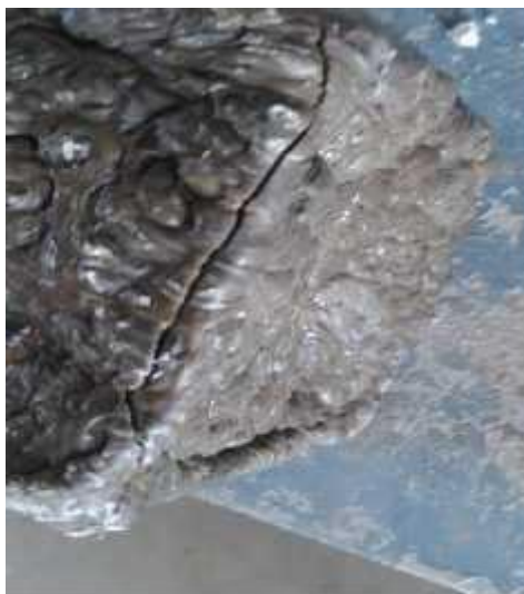
Figure 3.3 Stage of Failure
