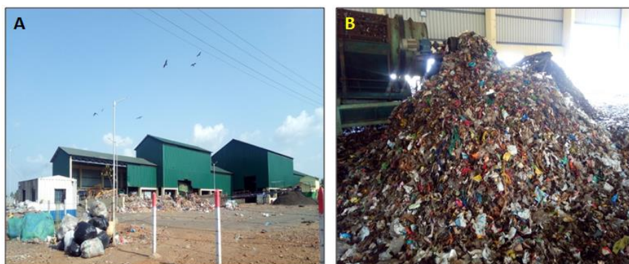
Fig. 17. A) Infrastructure of RDF Plant B) Final RDF
