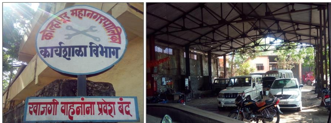
Fig. 11. Operation and Maintenance Facility of KMC
