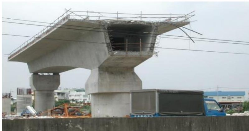
Figure 1: Box Girder Bridge [4]
