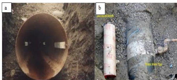
Figure 5. (a) Internal protection of water pipe-line using sacrificial anodic method (b) External protection of water pipe-line using sacrificial anodic method
