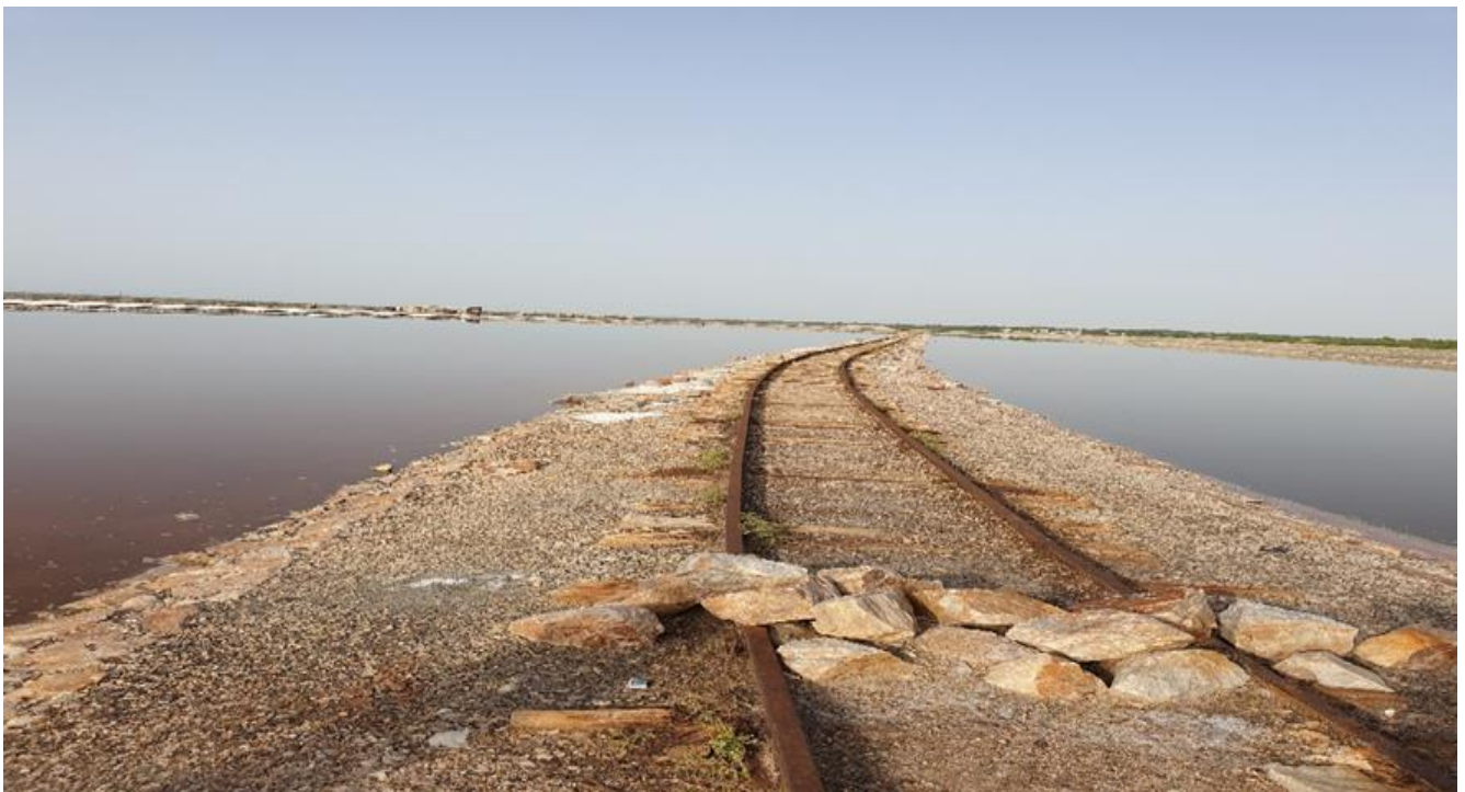
Figure 3 Trolly Rail line for transportation
