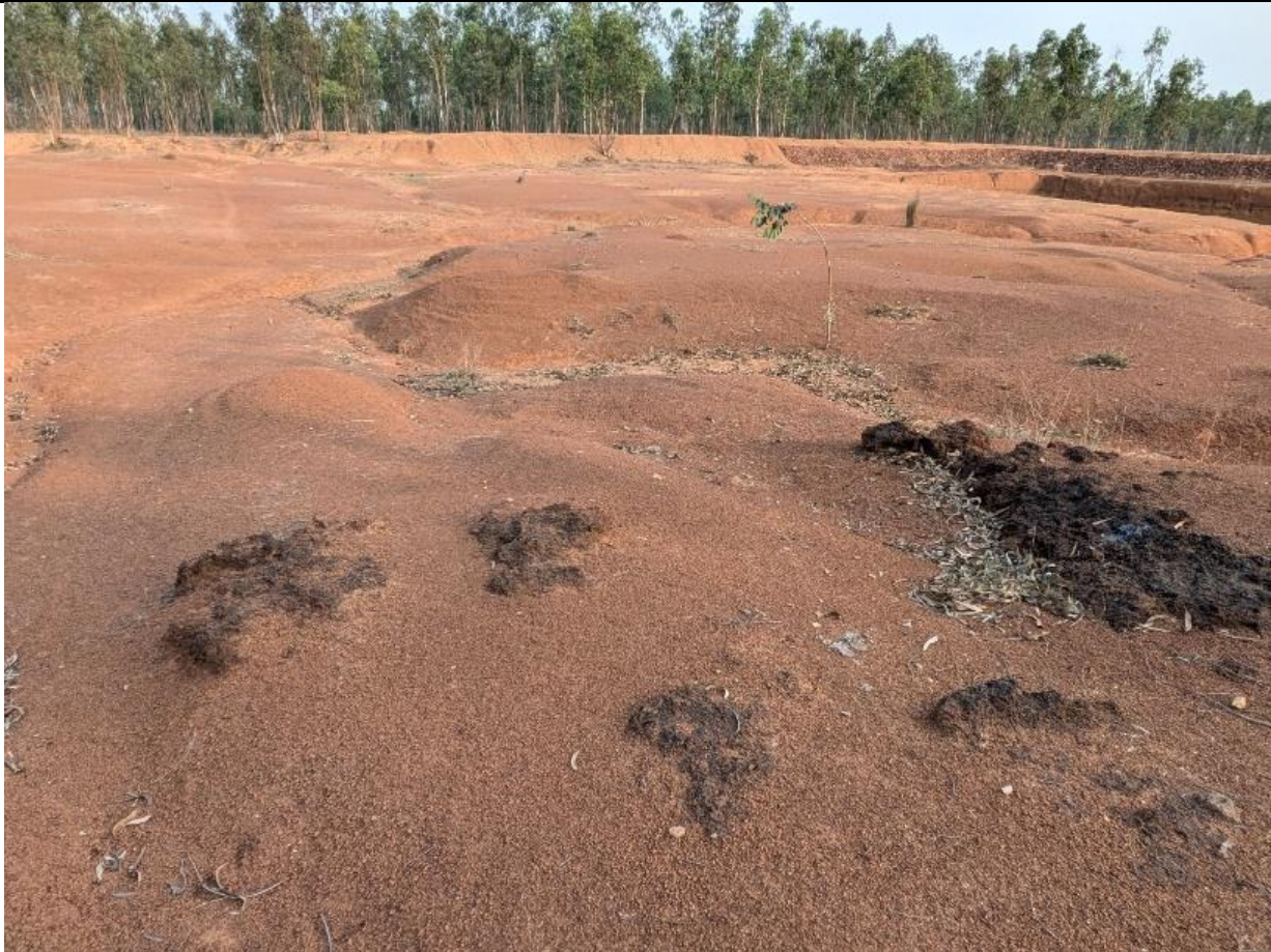
Figure 13: Surface Erosion Accompanied by Burnt Patches of Laterite Duricrust. This image illustrates sheet erosion and minor rill formation on a relatively level lateritic surface. The dark patches signify burned vegetation or biomass, potentially resulting from shifting cultivation, fire clearing, or human activities. These incinerated areas may further expose the soil to erosion, thereby exacerbating the loss of topsoil. In the background, a sparse tree line delineates the transition between degraded land and semi-natural forest or scrubland.
