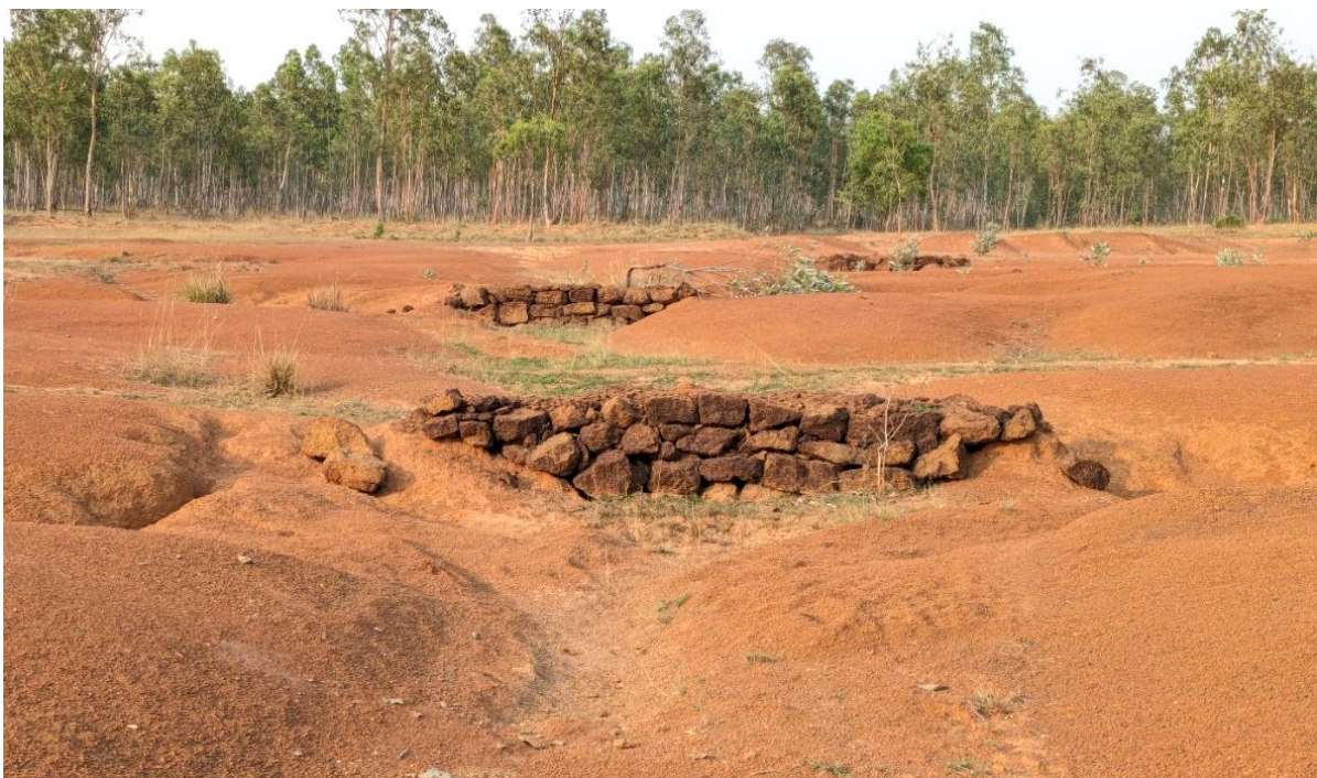
Figure 15: Construction of a Check dam on the main gully channel by using blocks of hardpan to reduce soil erosion.
