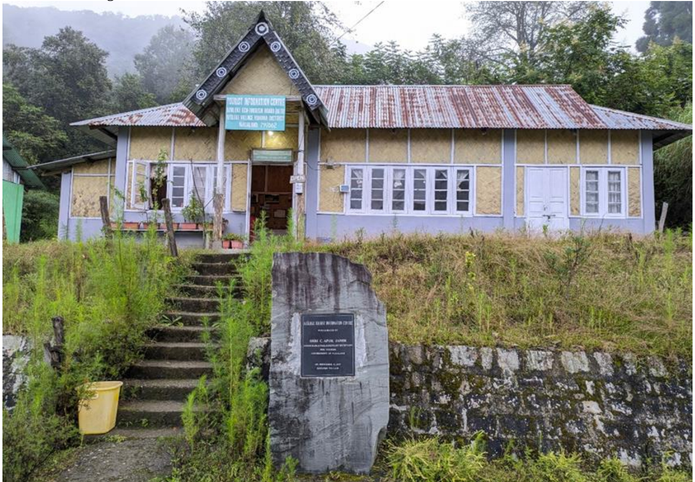
Figure 09. The photograph showcases the Tourist Information Centre of Dzuleke Village. The traditional sloping roof of the tin house and bamboo, mud-plastered walls represent the indigenous household pattern of Dzuleke. The building serves as a guide house for visitors. The signboard in this photo describes that this region is affiliated with the Department of Tourism of the Nagaland Government. It is a knowledge hub about local traditions, culture, customs, biodiversity, livelihood, and more. This image depicts their efforts to promote eco-tourism activities without interfering with ecological balance
