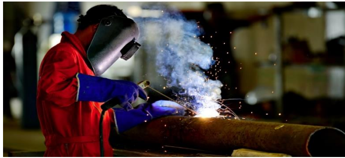
Fig. No. 17 Welding Safety
