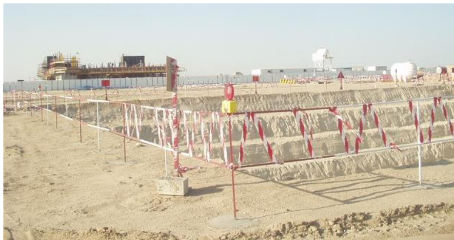
Fig. No. 09 Safe Baricade in Excavation
