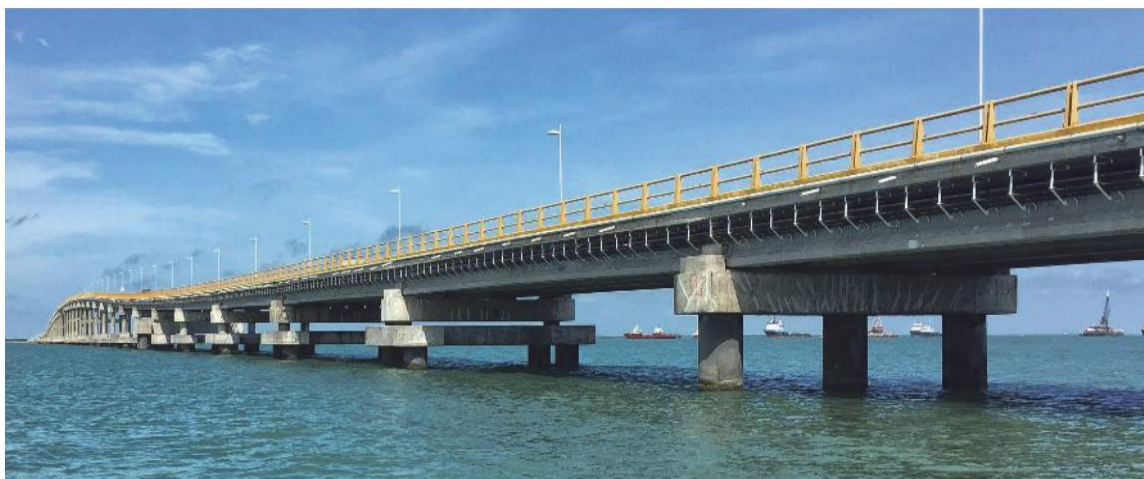
Figure 1.5: Bridge of pre-stressed concrete Girders el Zacatal, México [6].
