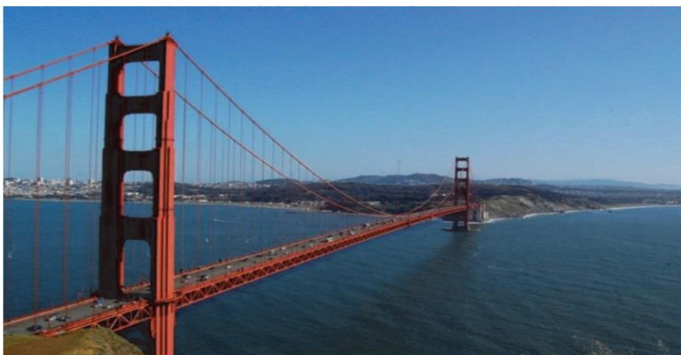
Figure 1.4. Suspended Golden Gate Bridge in San Francisco, California, U.S.A. [5].
