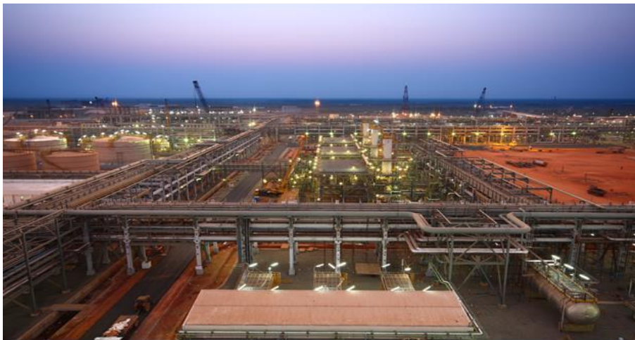
Fig 5.6 : Reliance Industries (RIL) Onshore Terminal at Gadimoga
