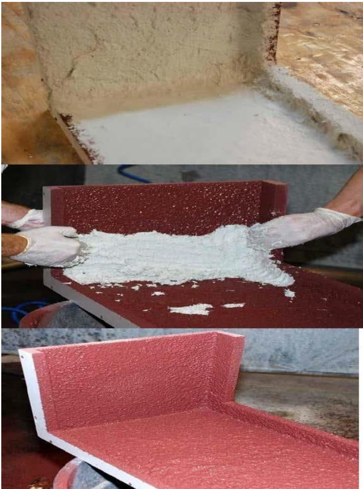
Fig. Hand packing backer on upright Fig. SCC backer in bottom
