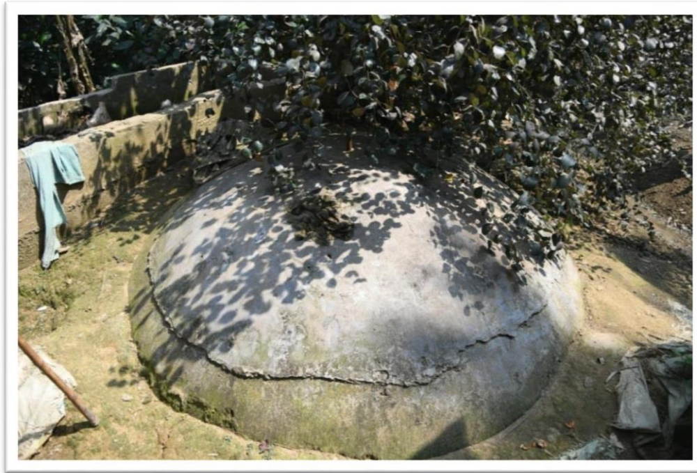
Fig 12: Bio-digester at Jorhat
