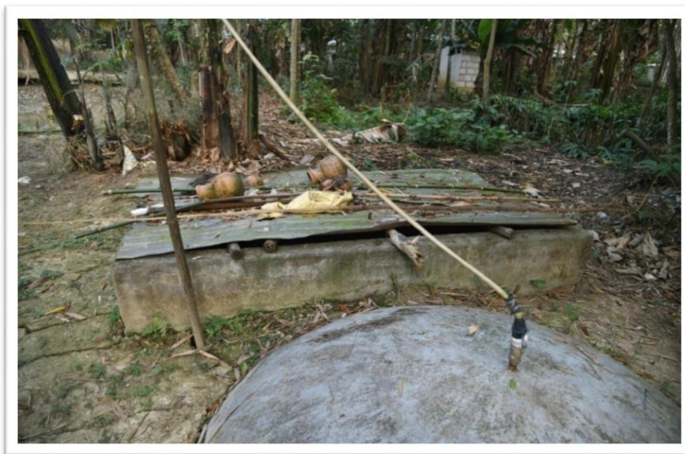
Fig 13: Bio-digester at Sivasagar
