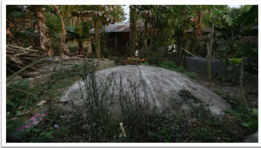
Fig 22: Abandoned Plant due to construction defect at Dibrugarh
