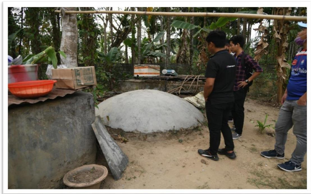
Fig 15: Bio-digester at Sivasagar
