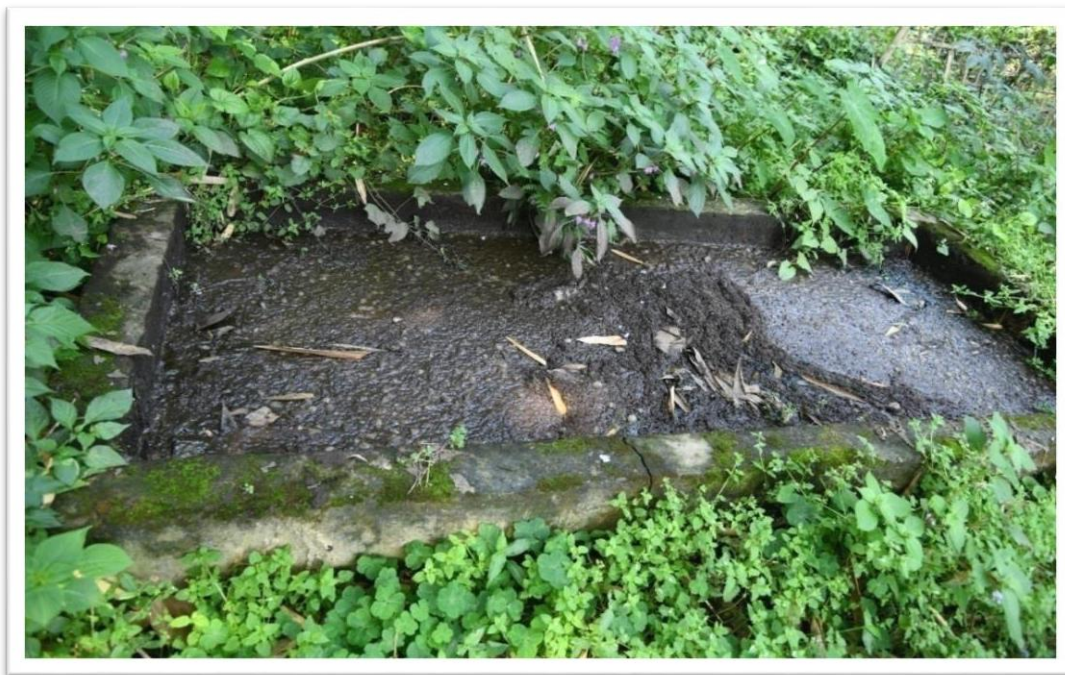
Fig 19: Slurry Pit at Sivasagar
