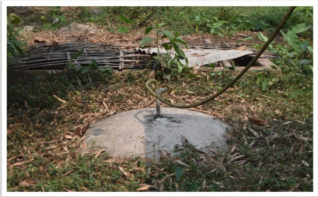
Fig 14: Bio-digester at Sivasagar
