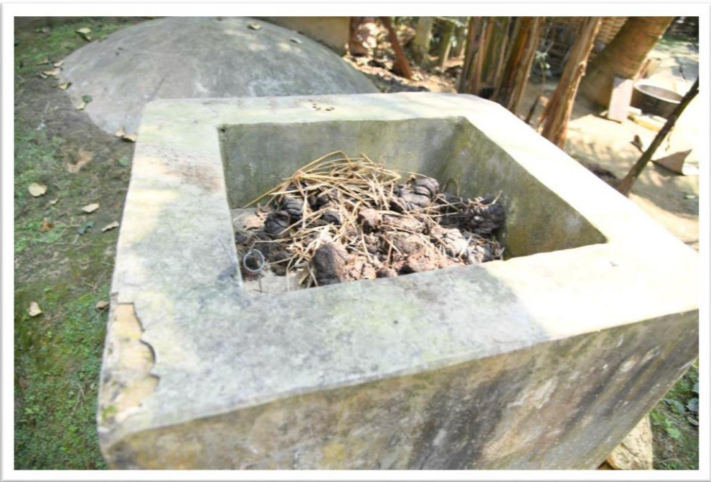
Fig 11: Slurry Inlet Tank at Sivasagar district
