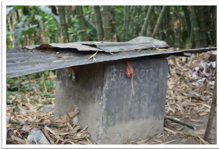
Fig 8: Slurry Inlet at a Jorhat rural residence
