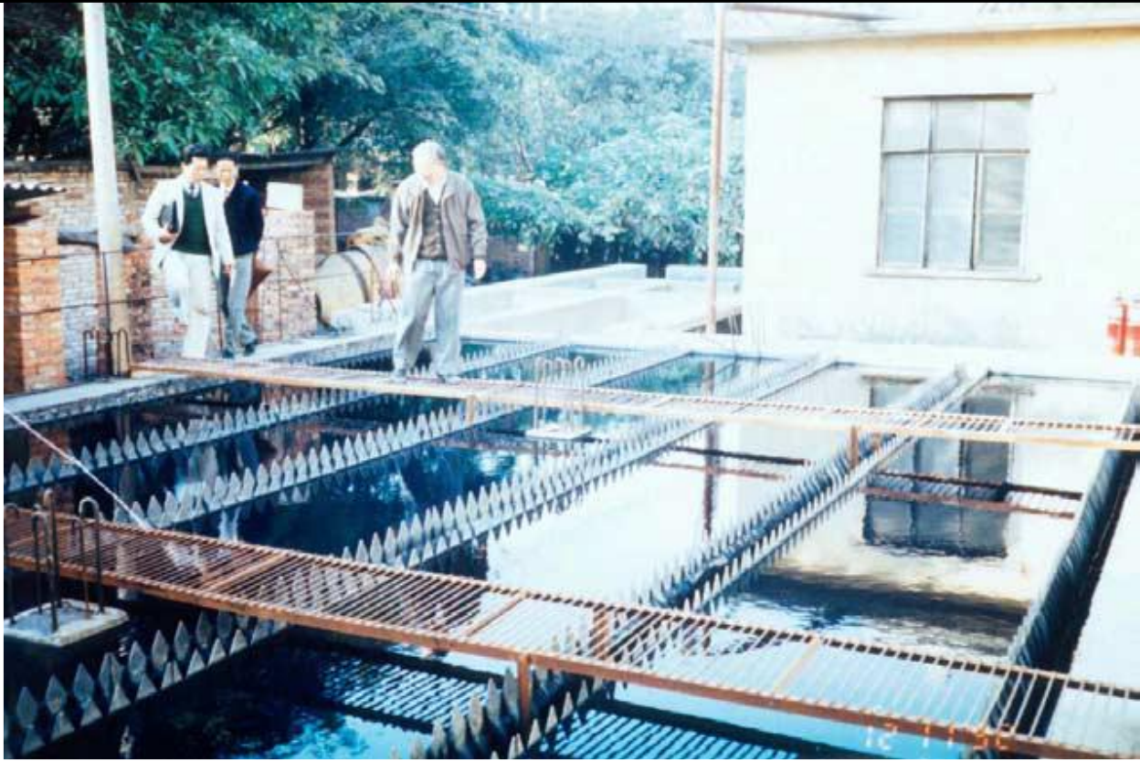
Fig. 4.4.4. Rectangular clarifiers follow coagulation/flocculation at a textile dyehouse. Rectangular
